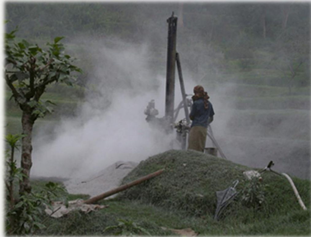
In Hills Blasting Rock Work
