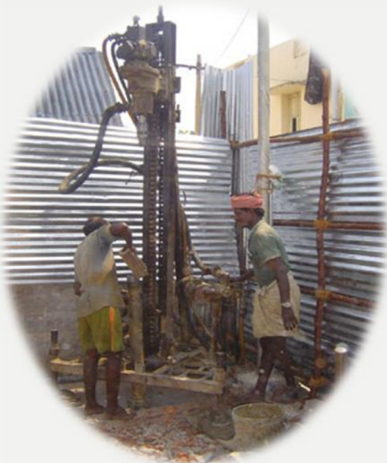
Small DTH Rig works
