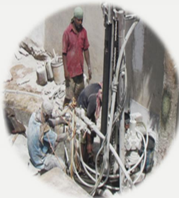
Handset Rig works
